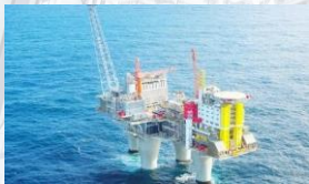
洋上への送電 Power from shore
