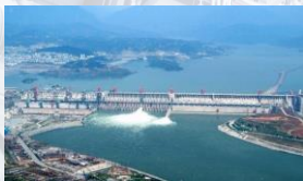
遠隔電源の送電 Connecting remote generation
