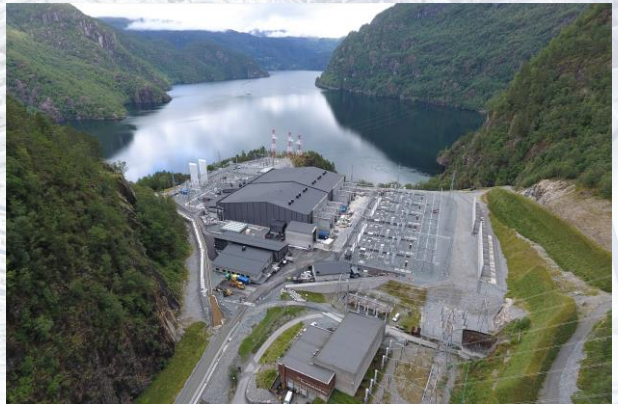
Kvittdal Converter Station (Norway)
