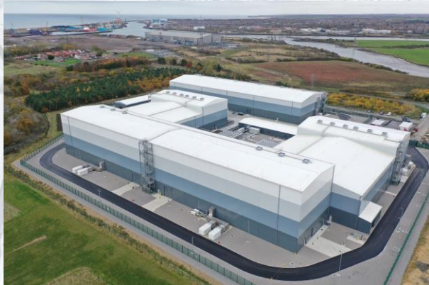
Blyth Converter Station (UK)
